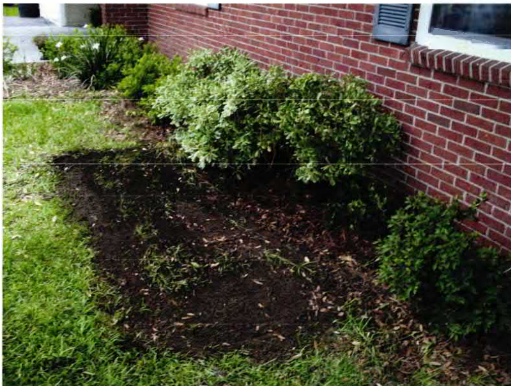
Picture 2: UST 862Dolphin excavation site after completion of work.
